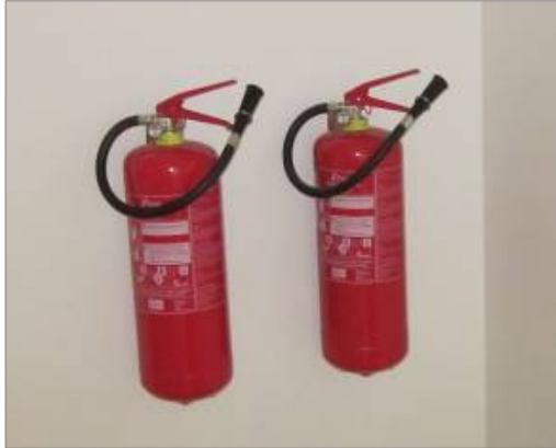
(6 kg dry chemical extinguishers)
